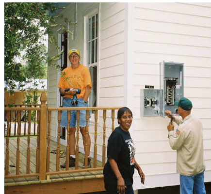
Homeowner Karen Keeve and volunteers as Katrina Cottage project nears completion.
