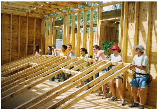
College students putting pre-framed wall in place on Katrina Cottage.
